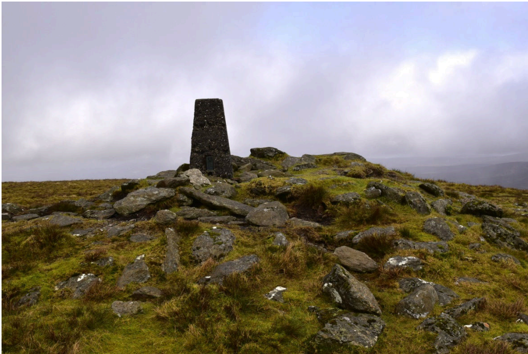
Figure 5. The triangulation pillar on Sawel sitting on a low cairn of boulders and peat that is probably the remnants of the 1827 OS cairn.
