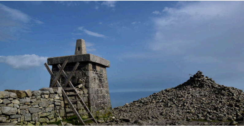
Figure 4. The triangulation pillar on Slieve Donard. The conical cap of the tower was removed to provide a flat surface for the pillar. The remains of the Great Cairn topped by the modern walkers cairn is to the right.
