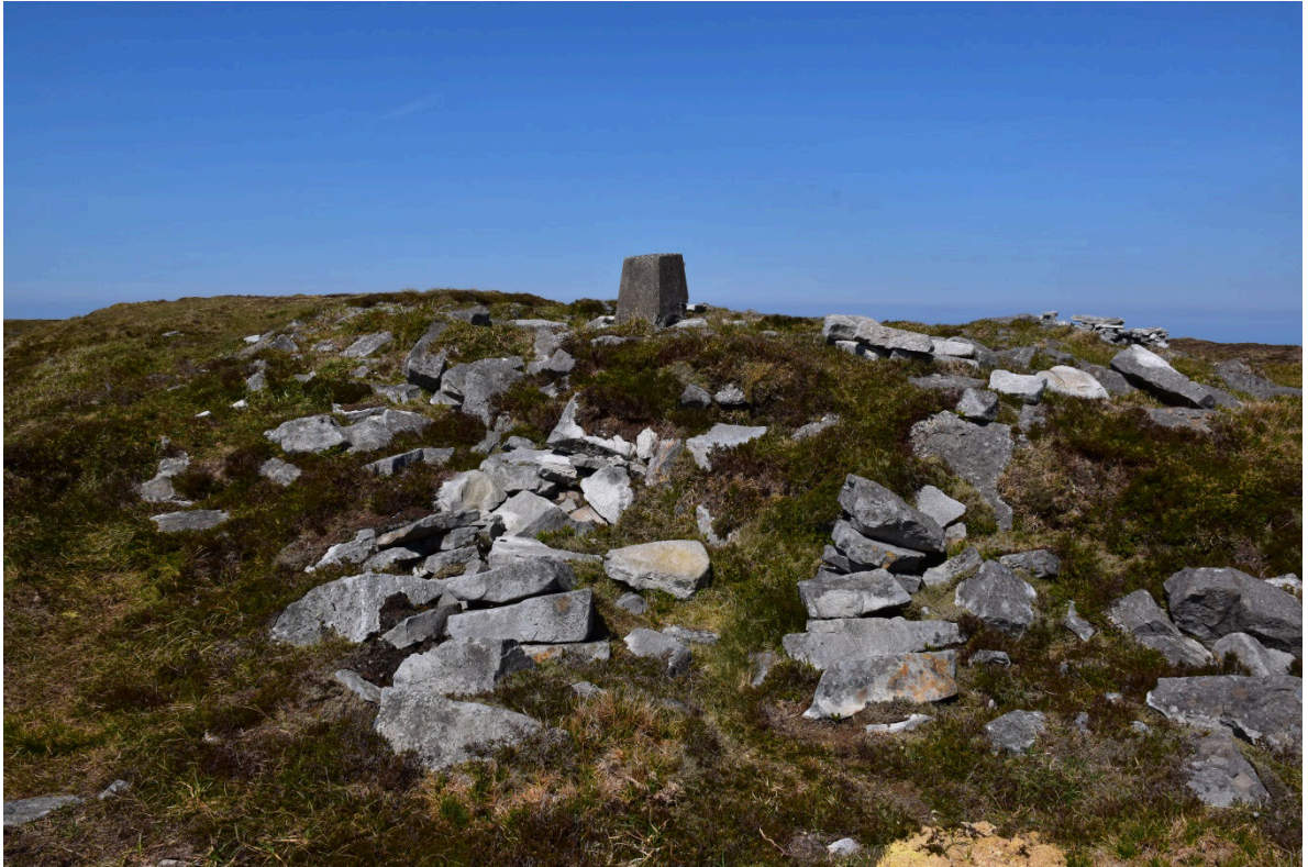
Figure 5. Slieve League summit with its slightly truncated triangulation pillar situated on the pile of stones that previously supported the 3-ft theodolite in the winter of 1827-28.
